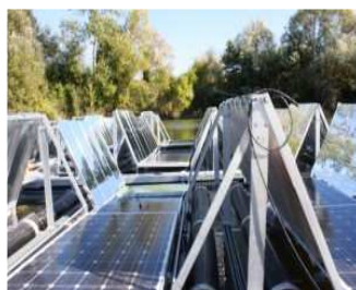
Concentrators in an FTCC plant. Photo by Scienza Industria Tecnologia.
